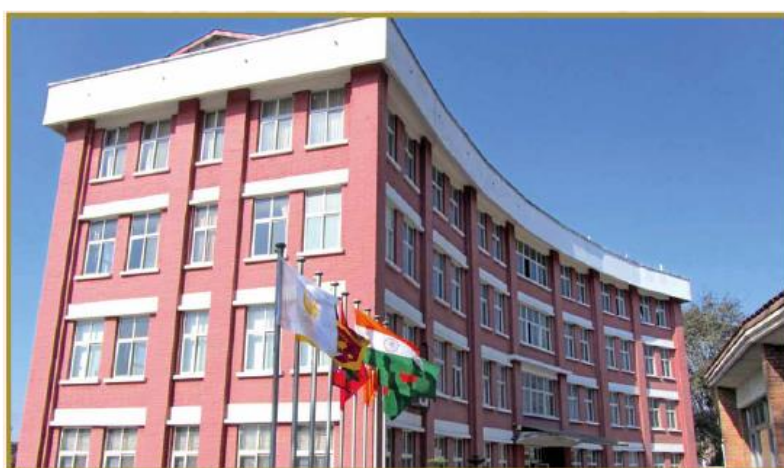
(Office Building of SAARC TB and HIV/AIDS Centre at Thimi, Bhaktapur, Nepal)
