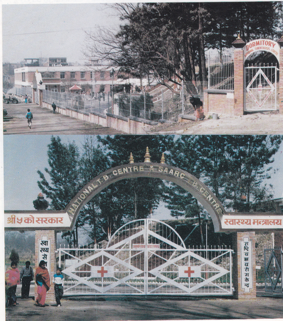
(Building of the SAARC TB Centre and National TB Centre)
